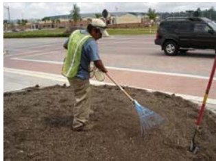
Step 2 – Clear Remaining Debris
